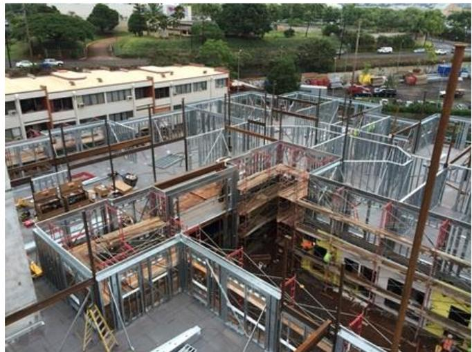
There was a stringent quality tolerance on the wall panels for the project to ensure precision in the framed structure. There were concrete shafts that needed to match the settlement with the framed walls along with structural steel members in select areas of the building, putting greater emphasis on panelization consistency. Group Builders chose CEMCO
